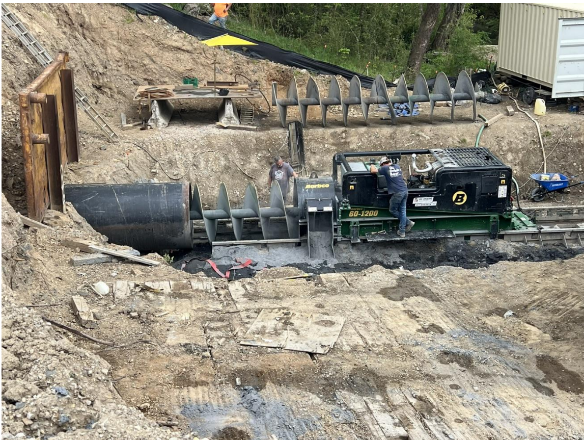
Boring under Malvern Avenue
