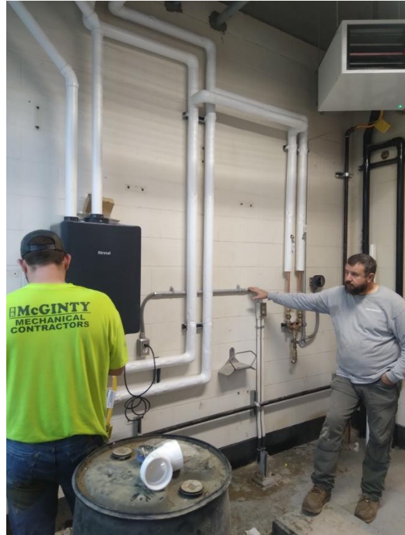
New Plumbing in Filter Building
