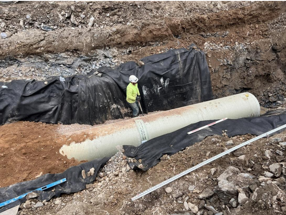
Gravity Main Construction
